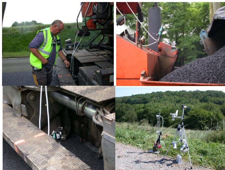
Photo 3 - Measurement points for fumes and dust and the weather conditions.
