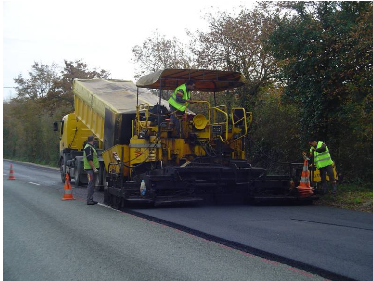
Photo 1 - Works on the RD 2160, laying train
