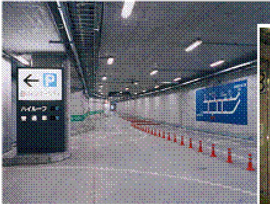
Large-scale underground driveway
