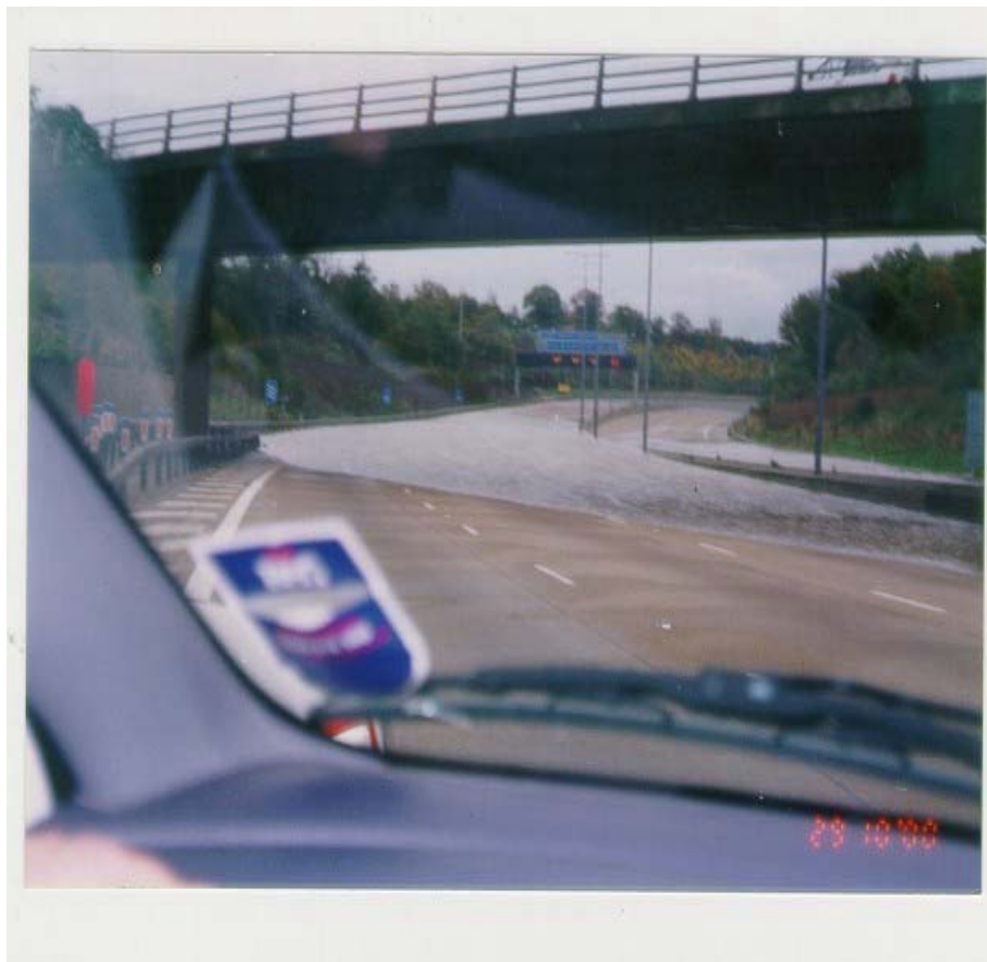
Flooding on M25
