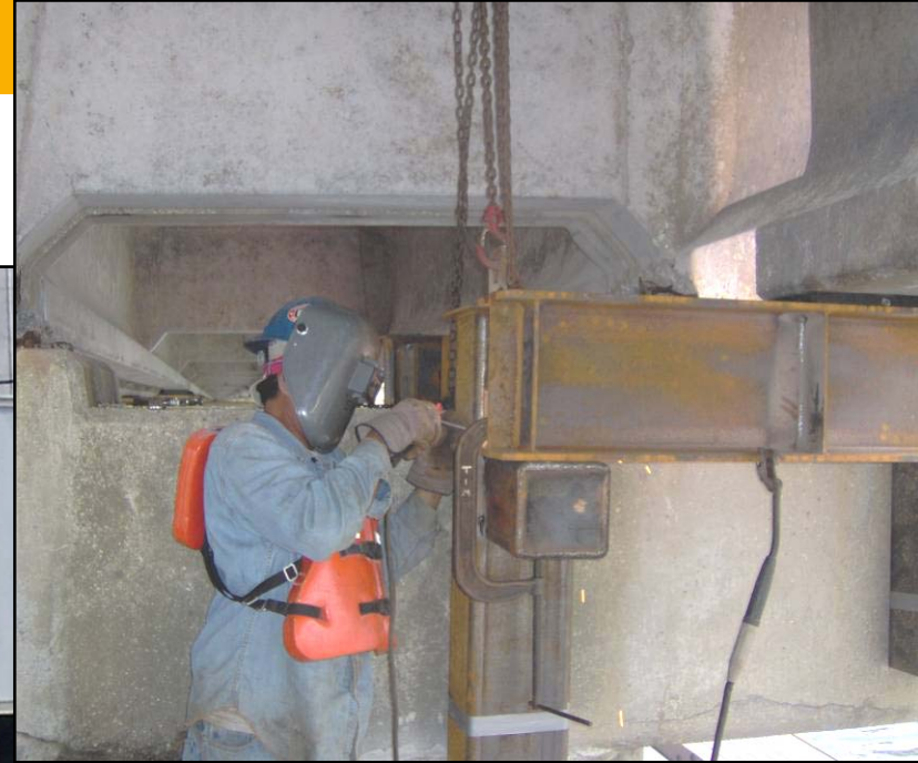
Inspecting the bridges
