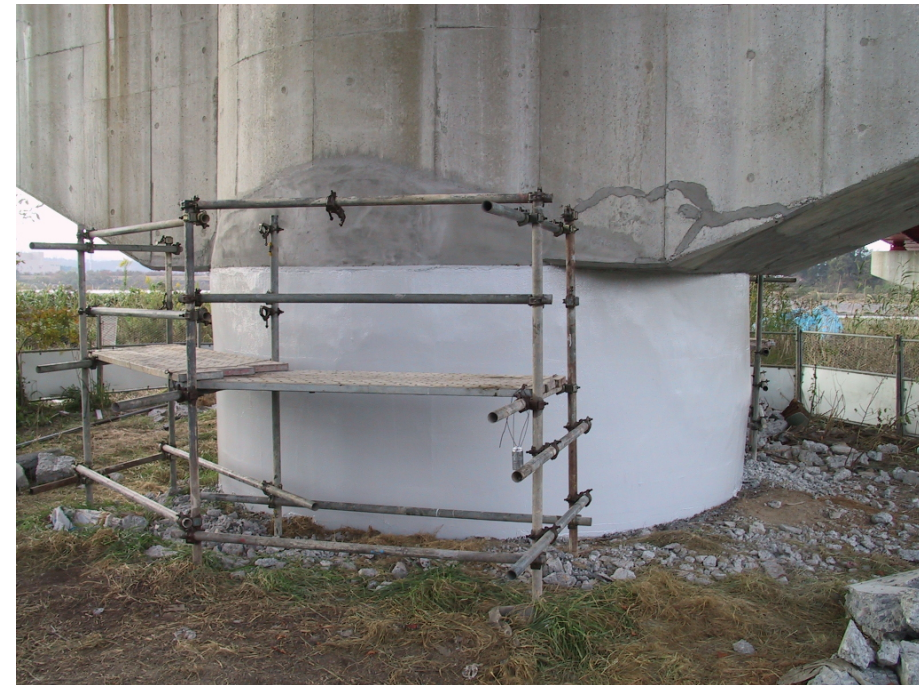
Emergency Repair by Carbon Fiber Jacketing
