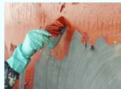
Newly developed removal method※ (causing no scattering of paint coating film dust, noise or odors)
