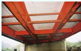
Existing paint coating
