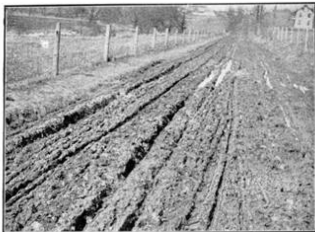
FIG. 143.—Section of Country Road before Improvement.
