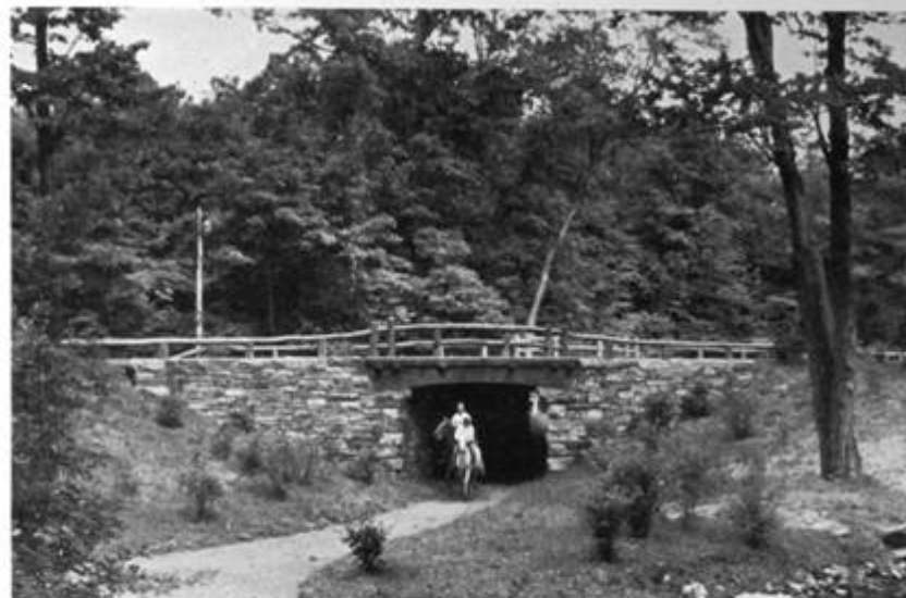
HUTCHINSON RIVER PARKWAY
