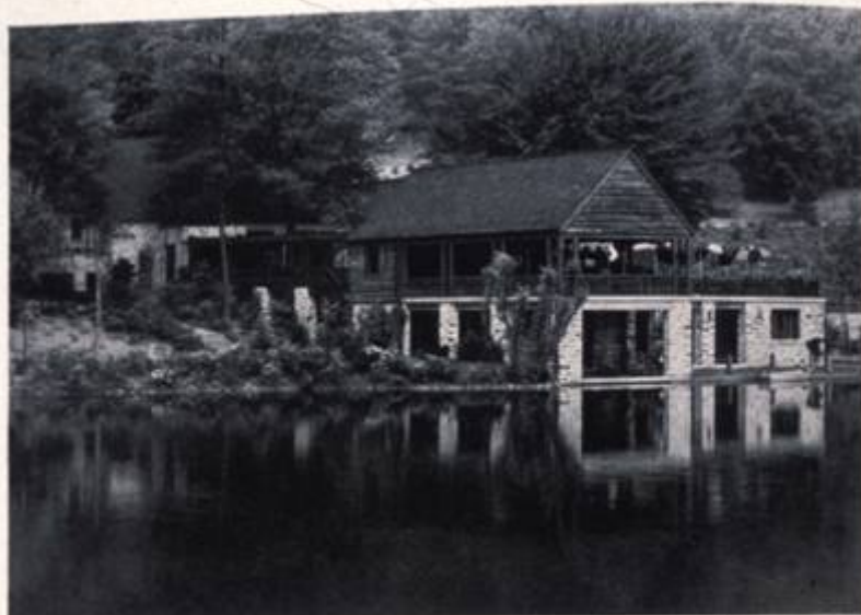
Restaurant at V. Everit Macy Park, Saw Mill River Parkway, Westchester County Park System Gilmore D. Clarke, Landscape Architect
