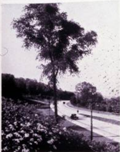
Roadbuilders have extended their vision beyond the edges of the pavement. In the development of highways in Westchester County, New York, the old limited ideas of roadbuilding have given way to new conceptions of landscape design, as may be seen in the accompanying views along the Sawmill River Parkway (above), the Bronx Parkway Extension (opposite, top), and the Hutchinsons River Parkway (opposite, bottom).
