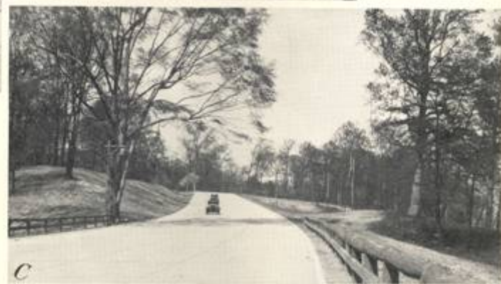
A. THE APPROACH TO WASHINGTON OVER THE OLD ROAD FROM THE SOUTH; B. VIRGIN TERRITORY WITHIN A SHORT DISTANCE OF THE FIRST PICTURE AND ON THE NEW LOCATION OF THE MOUNT VERNON MEMORIAL HIGHWAY. C. THE COMPLETED HIGHWAY AT SAME LOCATION NOW USED BY PASSENGER VEHICLES APPROACHING WASHINGTON.
