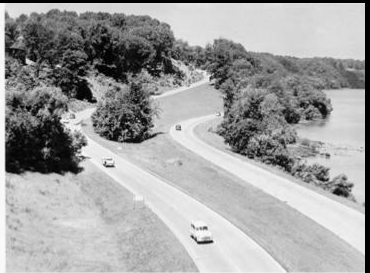
(50) The George Washington Memorial Parkway, an example of superb marrying of the road to the landscape. By running roadways independently, grading is kept to a minimum.
