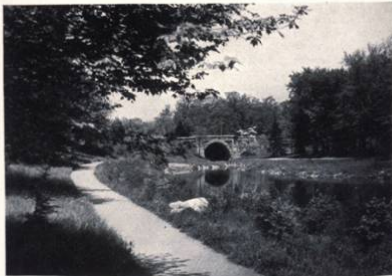
Underpass Bridge for Bridle and Foot Path, Hutchinson River Parkway, New Rochelle, Westchester County Park System
