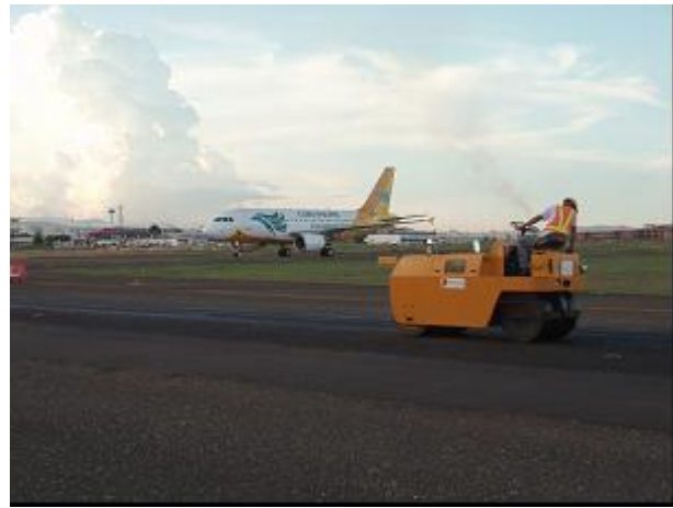
7.4 – Rolling/Compaction
