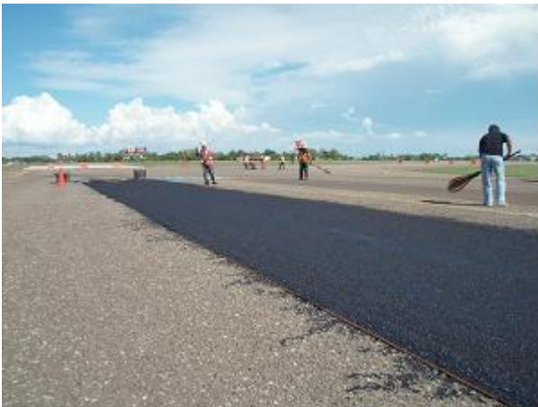
7.1 – Preparation, surface sweeping
