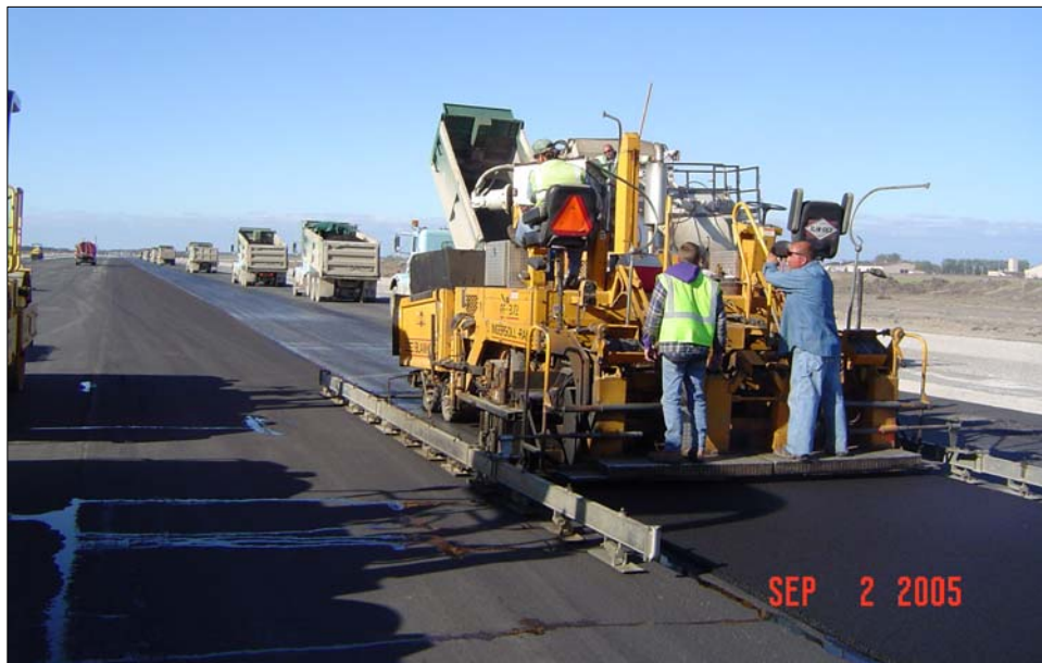
Figure 11. Placement of New Asphalt Surface
