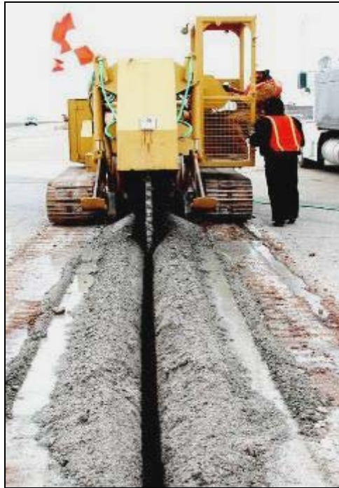
Figure 4. Relief Trench Cut with a Wheel Saw
