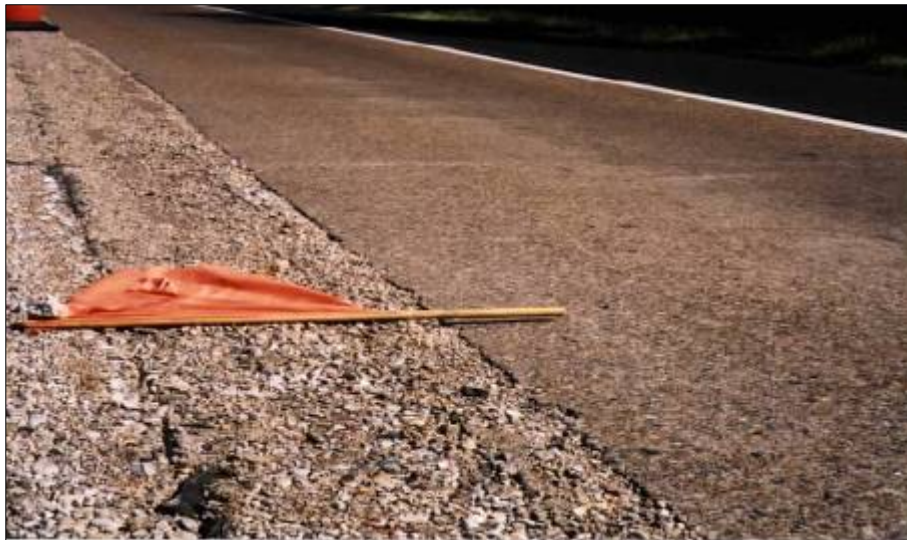
Figure 3. Vertical Displacement Prior to Rolling
