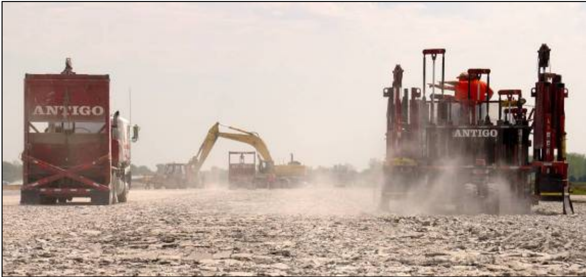
Figure 8. Dust generated during Rubblization
