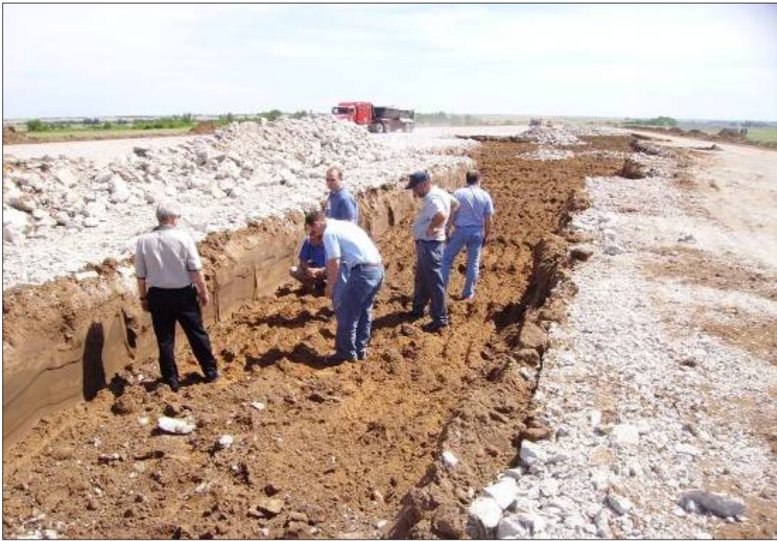
Figure 14. Full-depth Excavation Deep Into Subgrade of Patched Area at Kegelman
