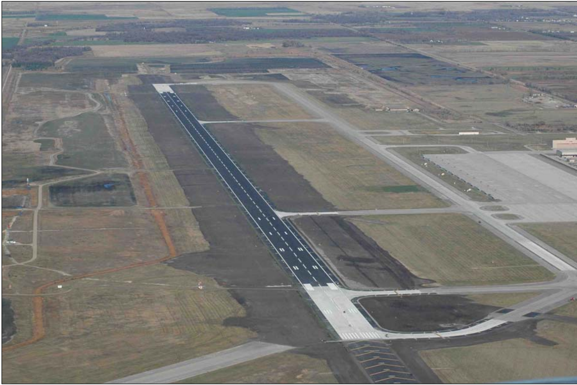
Figure 12. Aerial View of Completed Runway
