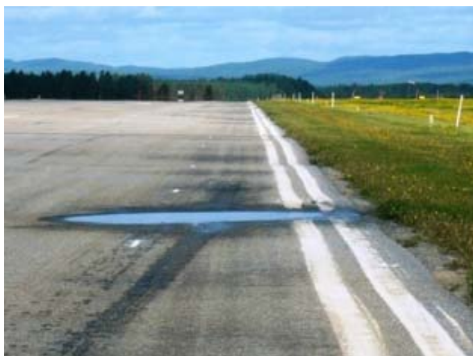
Figure 1 – Example of hazardous Runway unevenness
