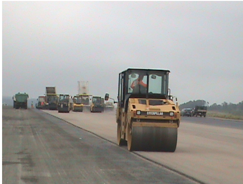
Figure 7 - Pavers and Rollers used on SMA Project.
