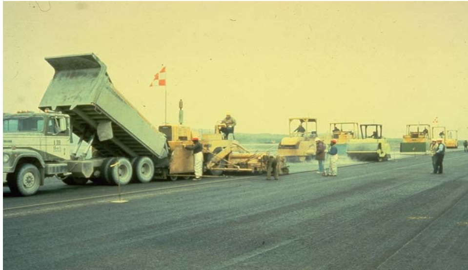
Figure 2. Placement and Compaction of 2-inch overlay.
