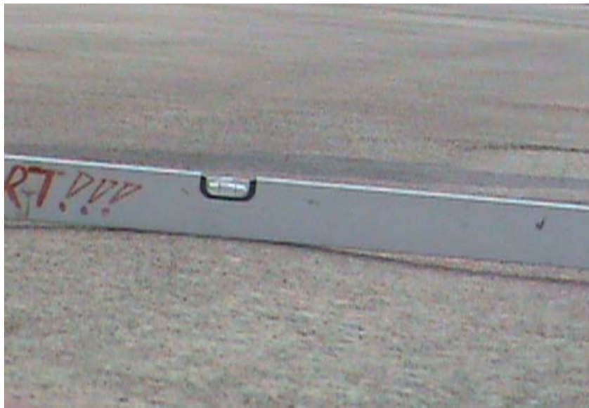
Figure 10. Blister caused by Water Vapor underneath the Pavement Surface.
