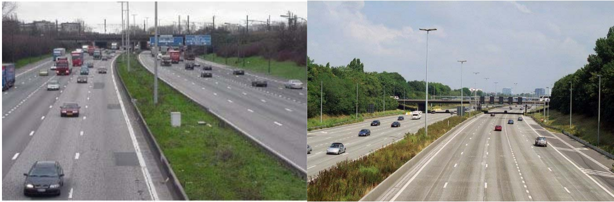
Figure 2 – Views on the Ring before and after the rehabilitation
