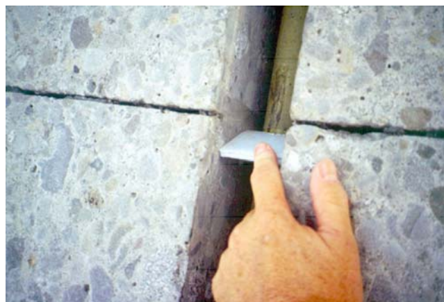
Figure 3 - Insertion of a spacer into a slot with dowel bar.
