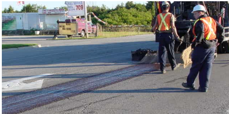
Figure 9 - Pre-treating of moderate alligator cracking at the centerline.
