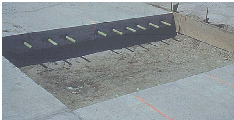
Figure 6 - 2 m repair area prepared for concrete placement.
