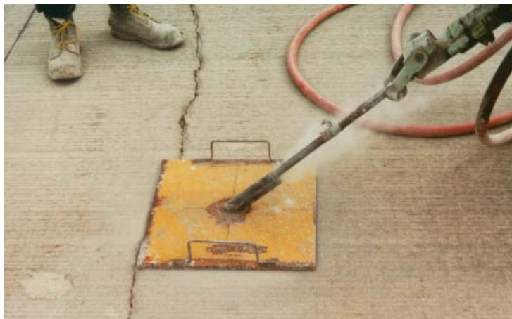
Figure 4 - Drilling holes for cross stitching.
