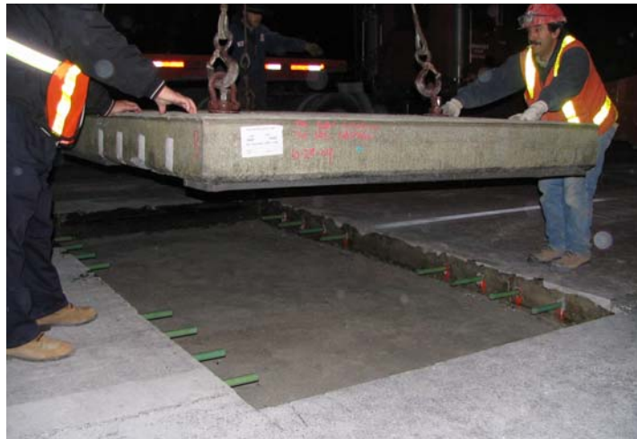
Figure 1 - Installation of pre-cast slab.
