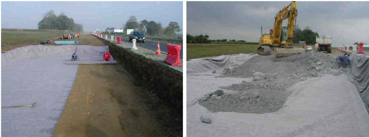
Figure 6 - implementation of the sealing and the MSWIA – RD767 instrumented roadway
