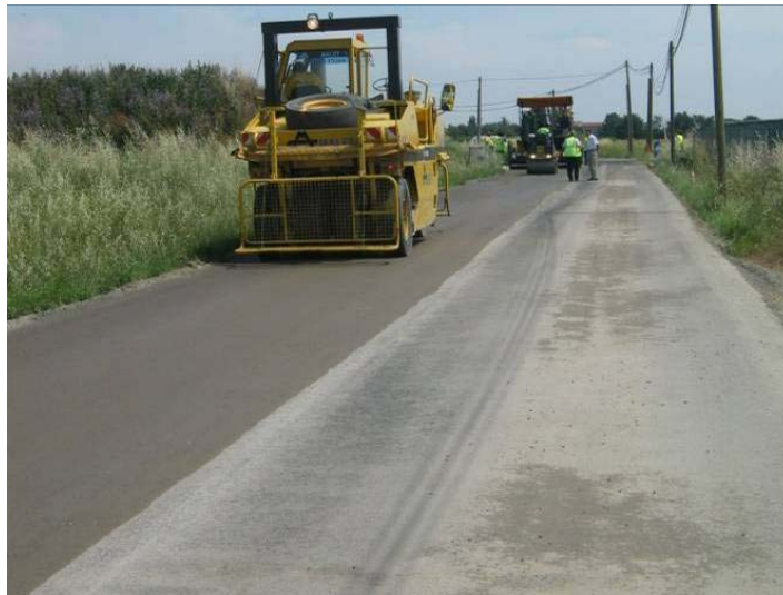
Figure 7 – Application on site by half road width
