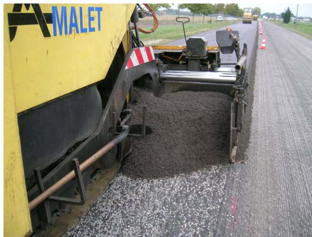
Figure 9 – Application on site by half road width
