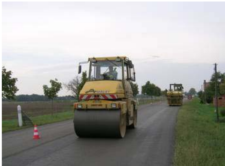
Figure 10: Site compacting
