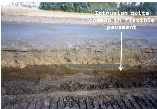
Figure 6 – Material intrusion
