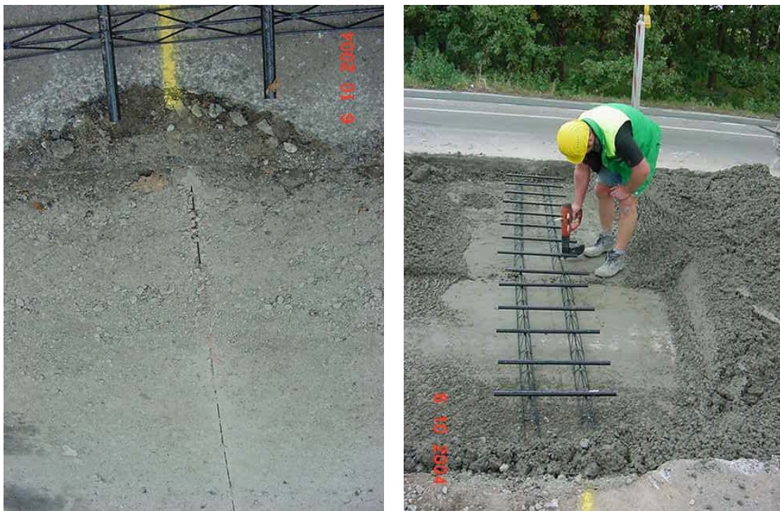
Figure 2 - Incision in the RCC for the transverse shrinkage joint
