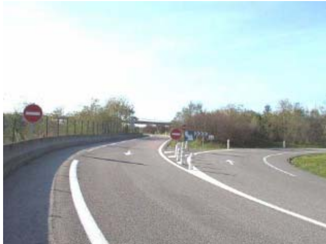
The B1 no entry sign and J5 directional marker in the diverging area are positioned side by side and arrows are marked on the road.
