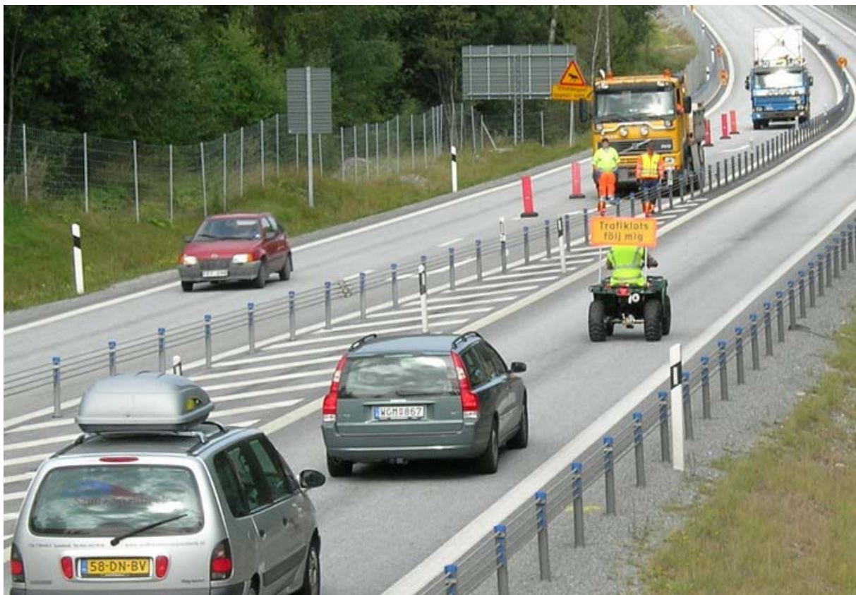
Figure 7 - Evaluation of a method to escort traffic through a work zone. This work zone is located on a road with a median barrier and alternating two traffic lanes in one direction and one in the other.
