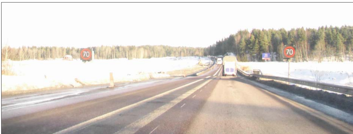
Figure 8 - LED sign in a sunny wintry landscape with the light from the side. In Sweden normal speed limit signs have been completely replaced by remote-controlled digital signs at a few roadworks. Observe the red border on the sign, which shows that this is more than just a recommendation. No evaluation comparing digital and traditional signs has been conducted as regards driver comprehension and the impact on speed. Some are of the view that it can often be more difficult to see digital signs than normal signs. Works executed by Vägverket Produktion at Västerås-Köping, February 2007.
