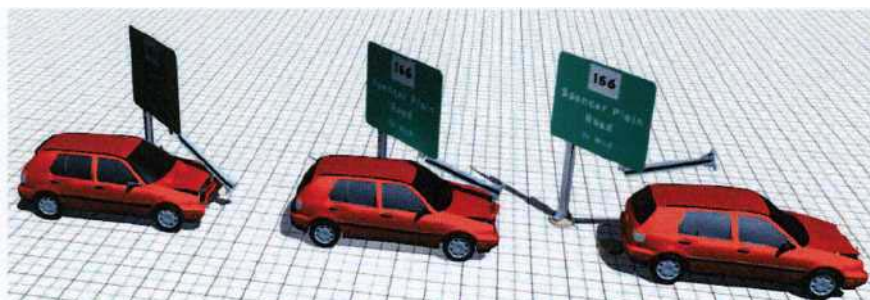
Figure 9 - Break-away roadside poles [7]
