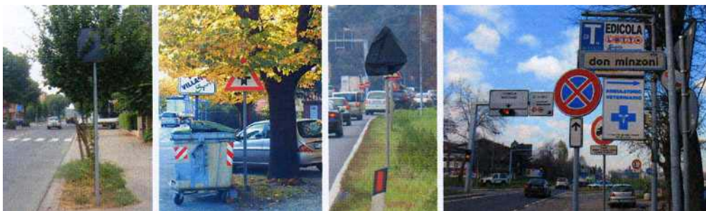
Figure 14 – Vertical signs not well perceivable by travellers
