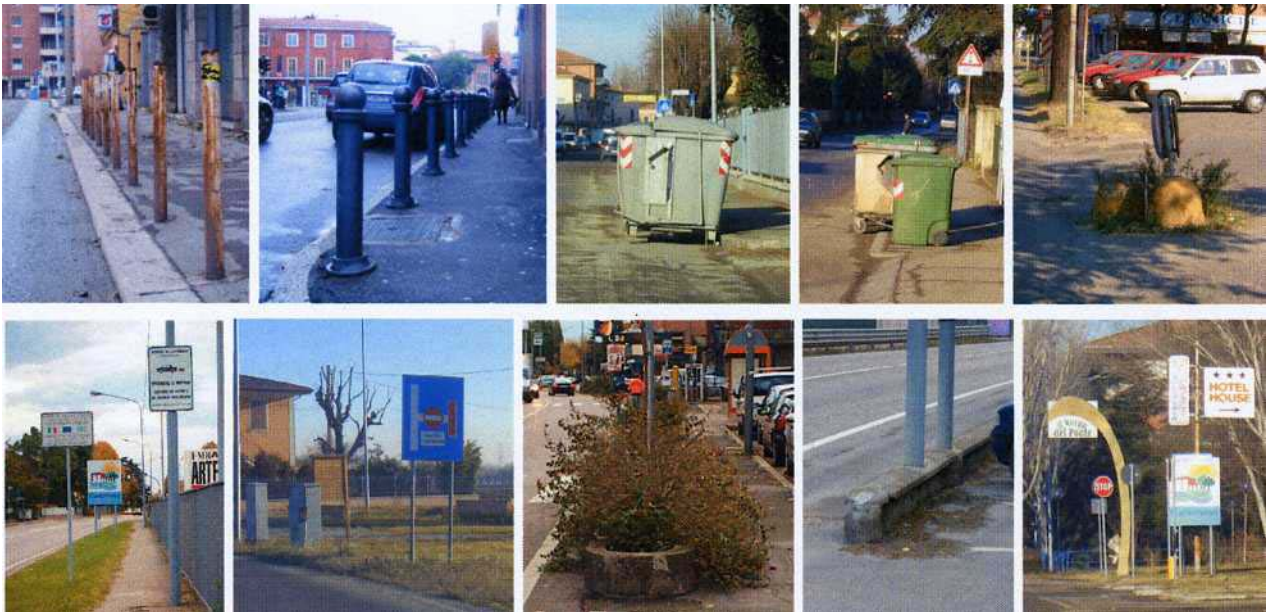
Figure 8 – Unprotected obstacles in shoulders
