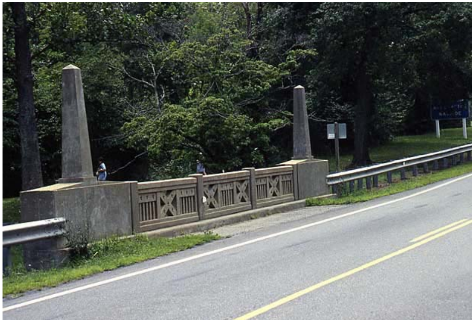
Figure 1 – Detail of concrete railing and obelisks, Appomattox County Structure No. 1002
