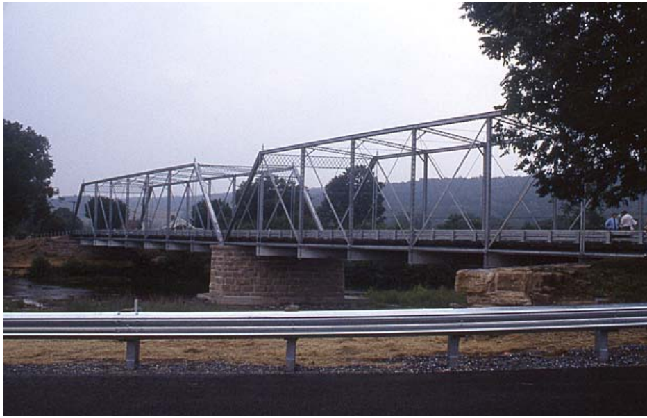
Figure 2 – The rehabilitated Goshen Bridge
