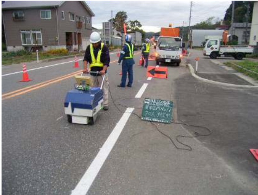
Data collection with a portable GPR
