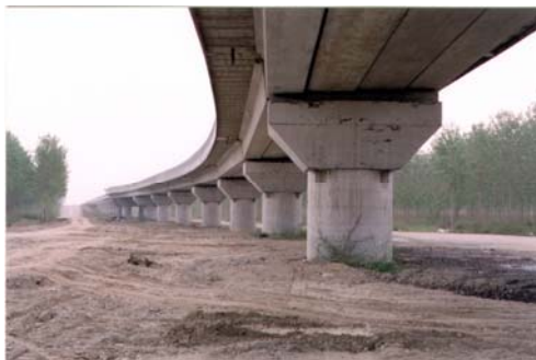
Photo n° 2 – The new viaduct of the main road 78 “Valenza – Rivellino”
