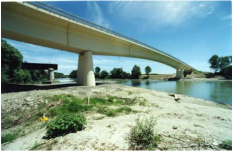
Photo n° 15 – The new bridge of Felizzano, with a view of the old structure in the background
