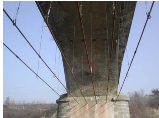
Photo n° 19 – Sight of the chains for 1° phase putting on safety.
