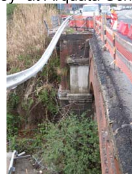
Photo n° 3 – The rebuilding of the pier of the collapsed bridge along the main road 140 “of Borbera Valley” at Arquata Scrivia
