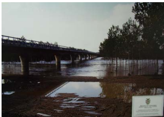
Photo n° 9 – The new bridge along the main road 87 – Static test made on 23/10/1999, in concomitance with the flood of the torrent Scrivia
