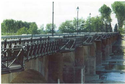
Photo n° 12 – The restored bridge, with its footbridge, in Castelnuovo Scrivia.
