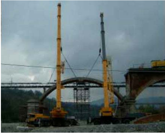
Photo n° 20 – Precasted semi-archs placed in yard.
