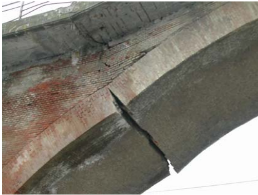
Photo n° 28 – Particular plastic hinge upon an arch
