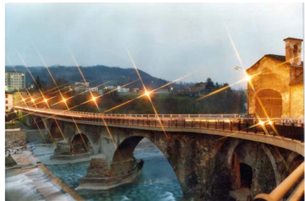
Photo n° 28 – General sight of the bridge on the Scrivia and of its footbridge / main road 143
