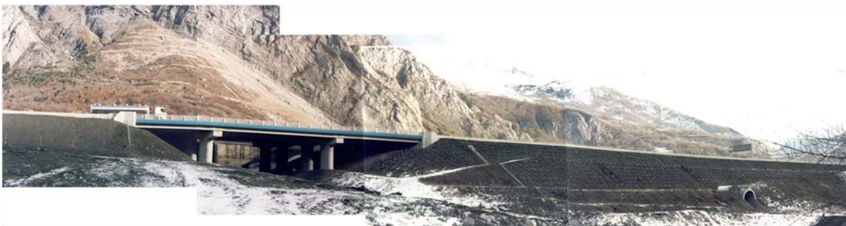
Figure 5: Structure OH90 in the Rieu Sec area (PI91 on the right).
