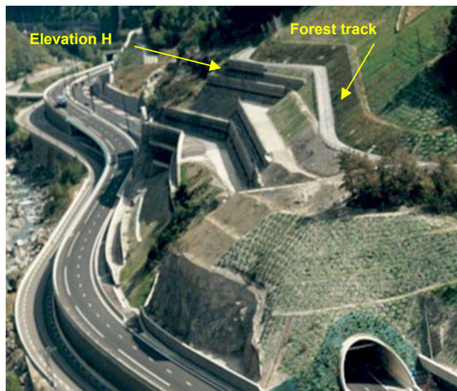
Figure 15– Locations of the measurement points on the retaining wall.
