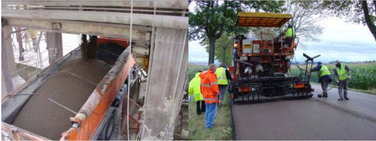
Photos 3 and 4 - Loading a truck at the manufacturing plant and laying the same mix on a very highly trafficked county road.
