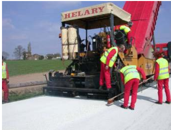
Photo 5 - Laying the white plant-based binder
