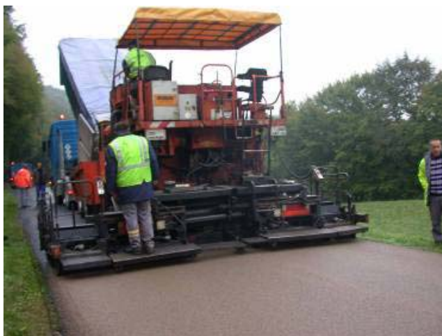
Photo 8 - October 2003, laying the 0/6 mix at Ligsdorf
