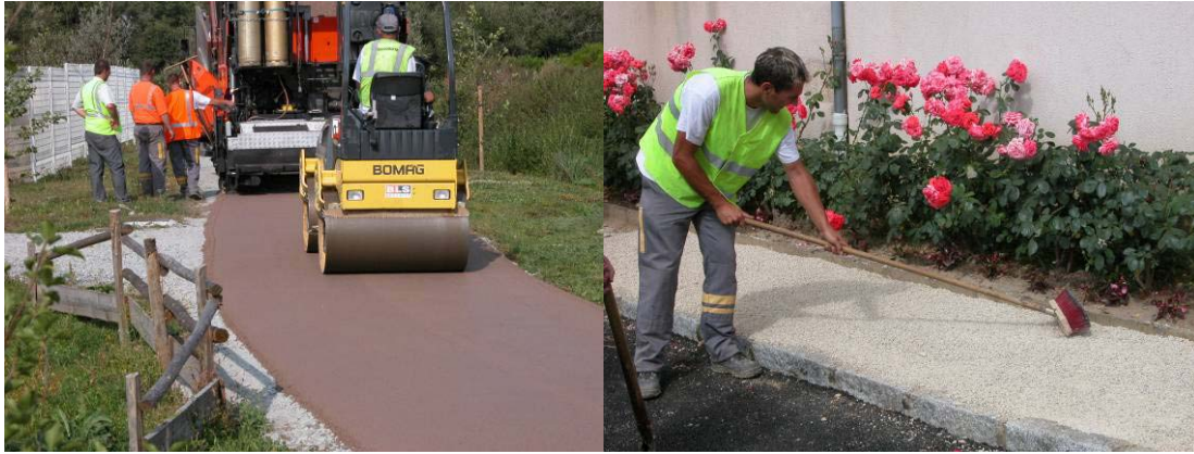
Photo 13 and 14 – Laying cold mixes manufactured with the plant-based binder emulsion.
