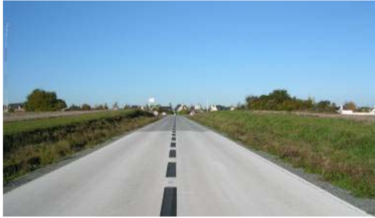
Photo 6 - Appearance of surface after cleaning with high pressure water.
