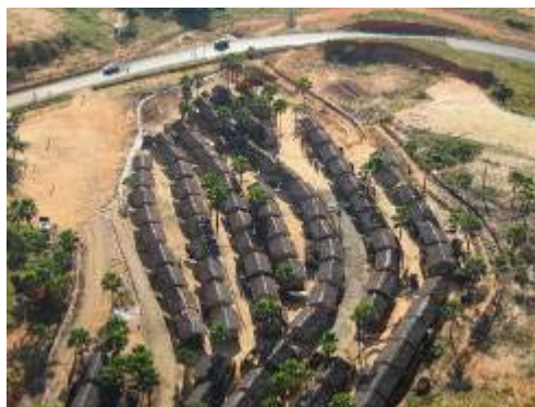
Figure 5 - Base vie ouvrière
