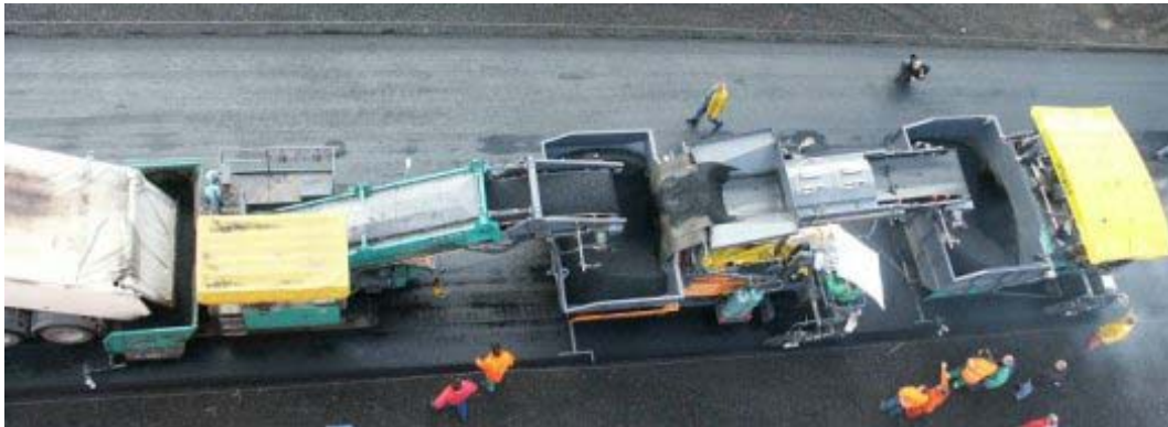
Figure 3 The laying operation with Process 2 using two finishers
