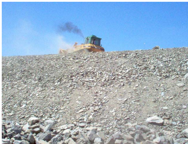
« Photo 2 – Sound schist from section 3 in embankments »
