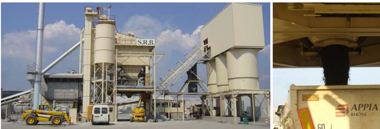
Figure 5. No fume emissions during the discharge in a truck at a batch plant.
