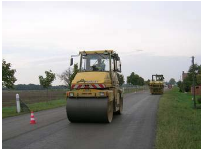
Figure 10: Compactage du chantier
