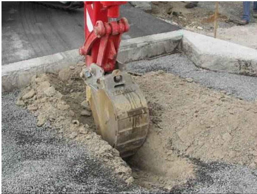
Figure 3 – Excavation of SECTM base course.
