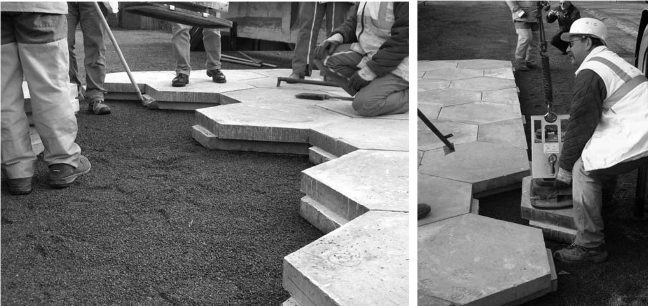
Figure 7 - The Autun solution (slabs with connection keys)
