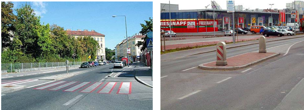
Picture 1 & 2: Red framed zebra crossing and Lane division
