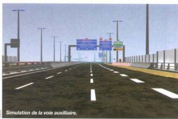
Photo 10 – General view of the concurrent section with the auxiliary lane
