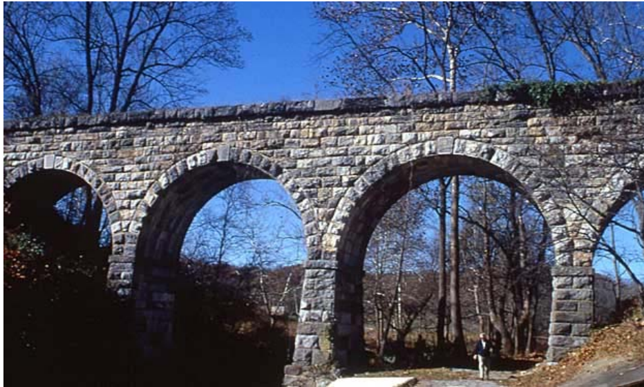
Figure 3 – Le pont Valley Railroad
