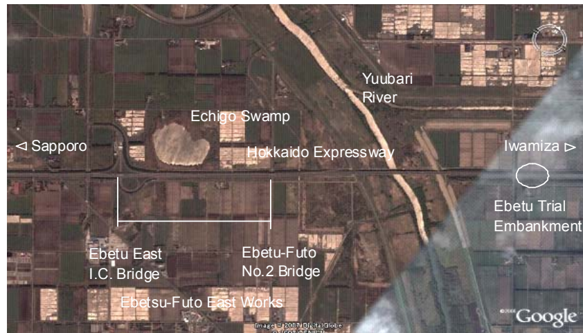
Figure 2 - The analyzed section in Hokkaido Expressway (©Google)
