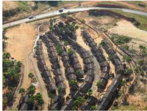
Figure 5 – Base camp for workers
