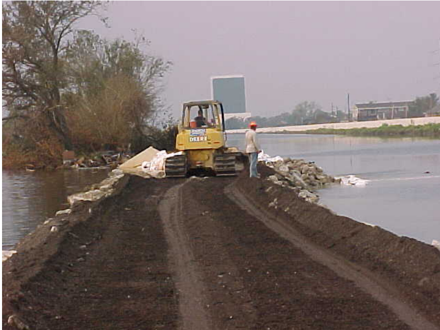
Figure 2 - DOTD crews build a road to facilitate levee repairs
