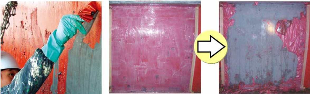
Photo 2 - Coating Film Removal Technology
