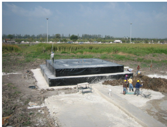
Photo 1 - Test Banking Construction
