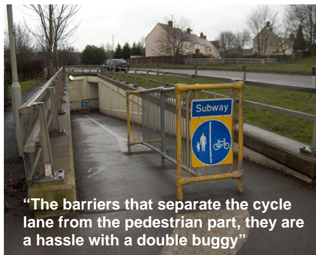
Figure 3 – Community perceptions of mitigation: subway entrance
