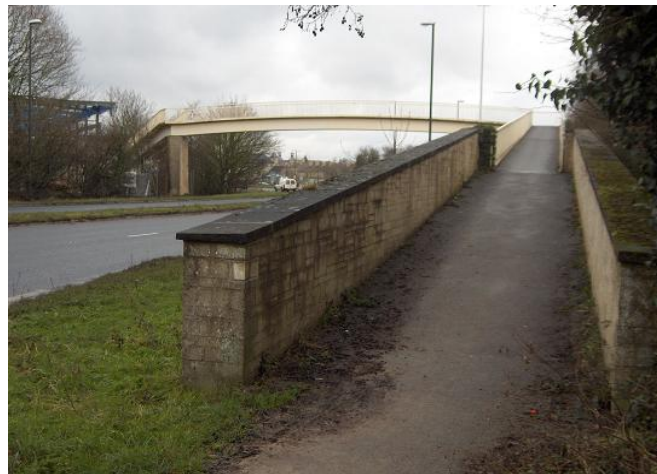
Figure 4 - Sloping ramp to footbridge
