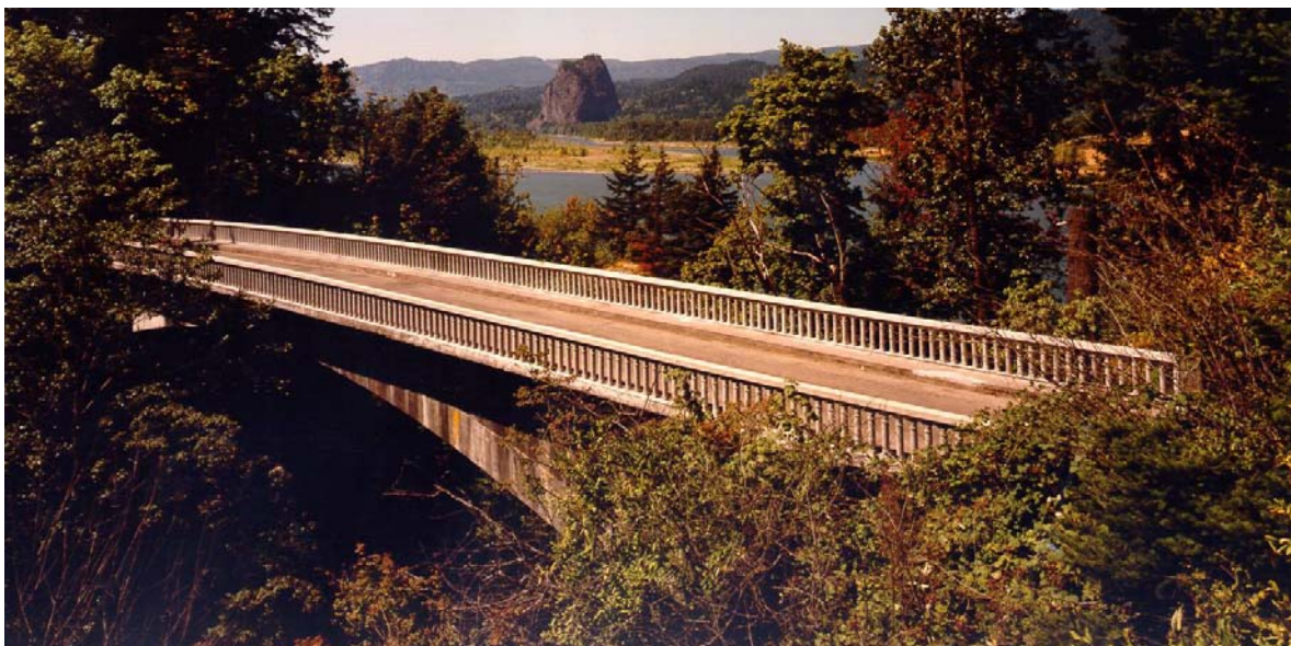
Photo 1—Moffett Creek Arch, Columbia River Highway
