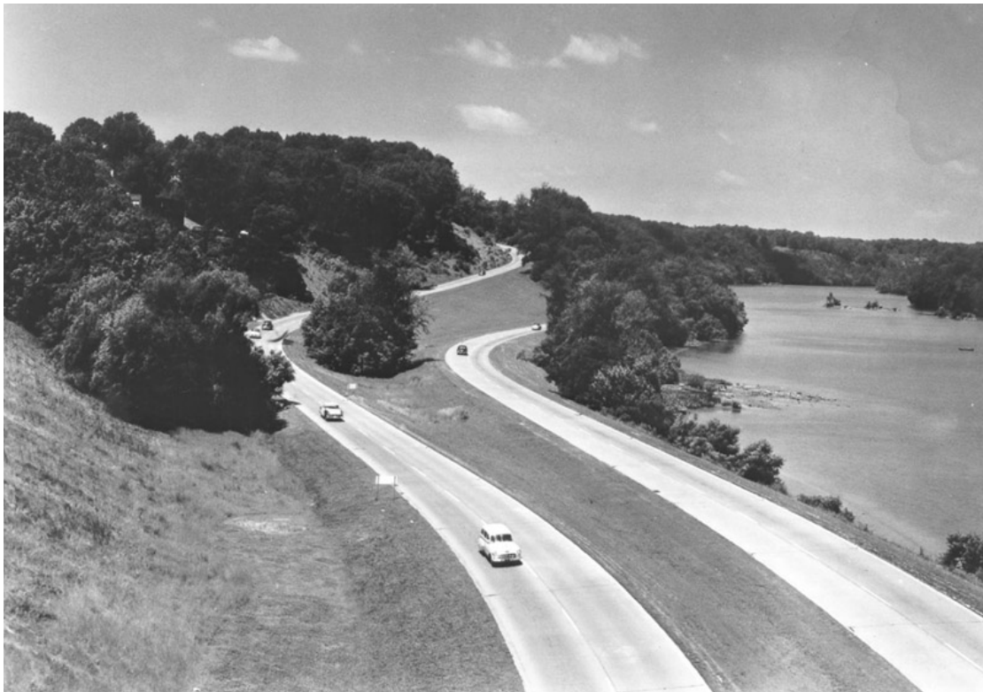
Figure-2 Postwar Section of George Washington Memorial Parkway, ca. 1955 (U.S. Bureau of Public Roads: National Archives)
