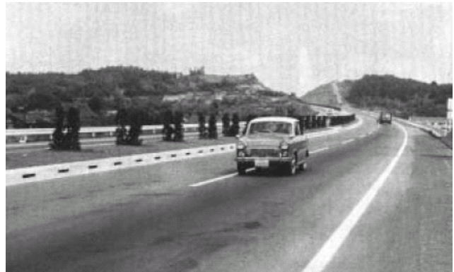
Figure 2 – First Expressway in Japan
