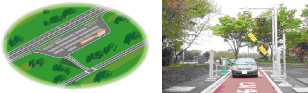
Figure 6 – Smart IC (ETC-only IC) placed on Parking Area
