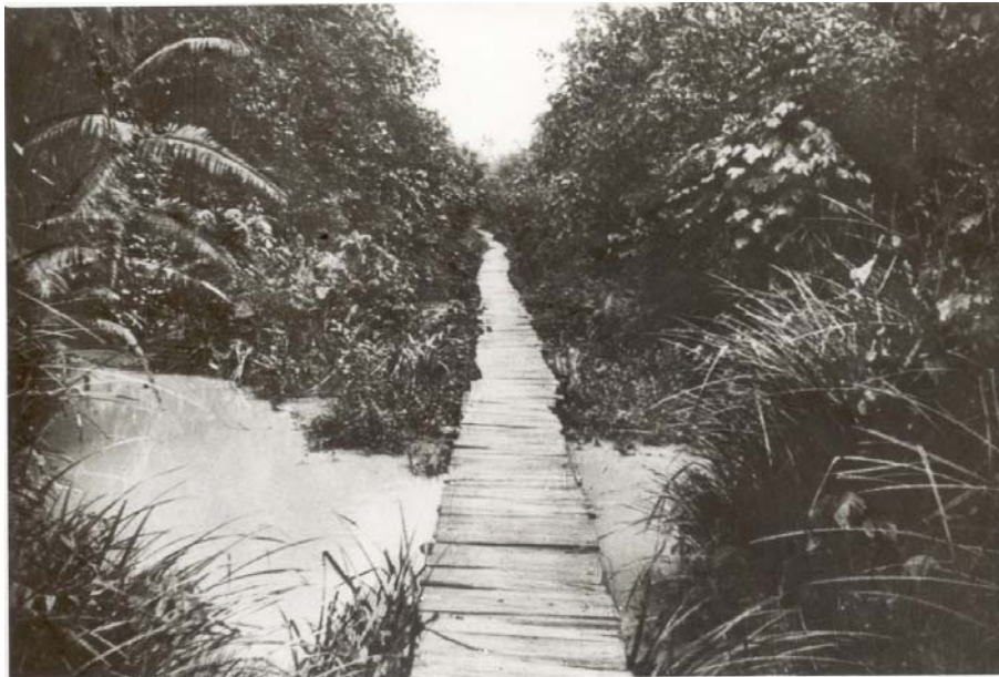
Photo 3 – Temporary bridge through swamp before Siamese military dig a big canal measuring 30 feet by 20 feet in depth to connect the two rivers, Jempol and Serting River.
