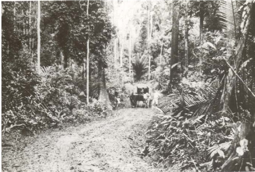
Photo 4 – Winding and bending road laid out for bullock-cart in order to consider the problem of animal traction and the importance of gradient.
