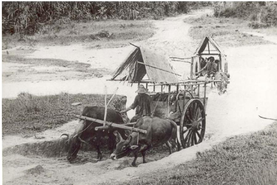
Photo 7 – Unsealed road performed well during dry weather but was hardly used by wheeled traffic especially bullock-cart in wet weather.
