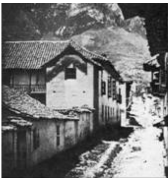
Remain silent of the observatory in Bogotá. System of evacuation of waters. 1842.
