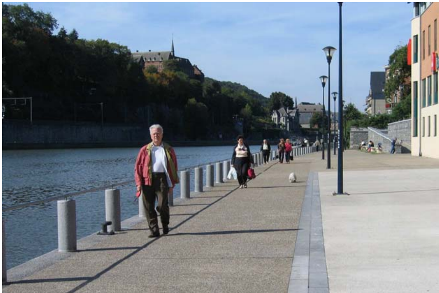
Figure 6 – coloured disactivated concrete (Dinant – Belgium)
