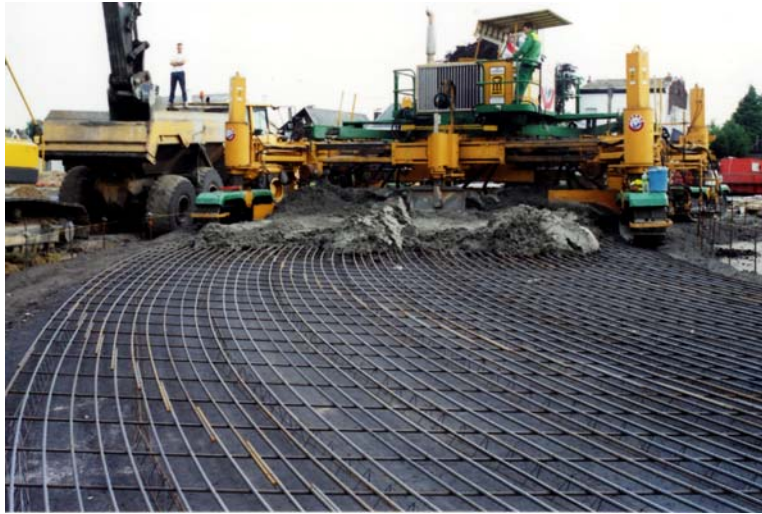
Figure 5 – Roundabout in continuously reinforced concrete
