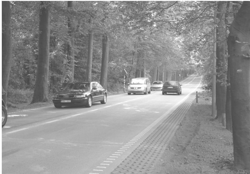
« Figure 4 – Overlay constructed in 2003 in the Drève de Lorraine, originally built in 1925 »
