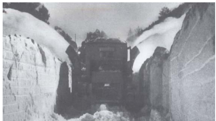
Fig. 12 and 13 AASS roadmen are re-plotting road on the mountain pass before re-opening it with rotary-type snow plough (1932)
