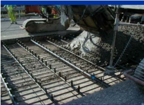
Fig 22 Eufonic Pavement with “canne d’organo” resonators
