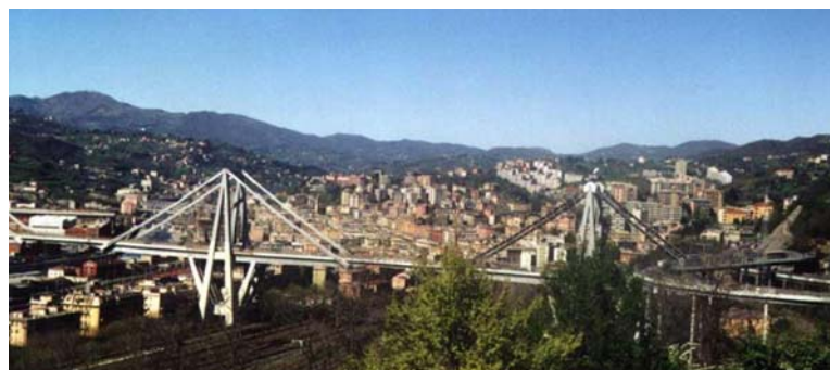
Fig.18 Vision of Polcevera Viaduct with new cables (right)
