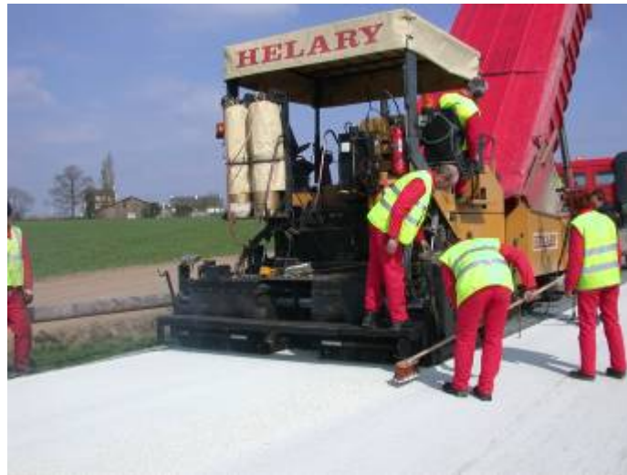
Photo 10 – Application of the very first asphalt mix using plant-based binder (white)
