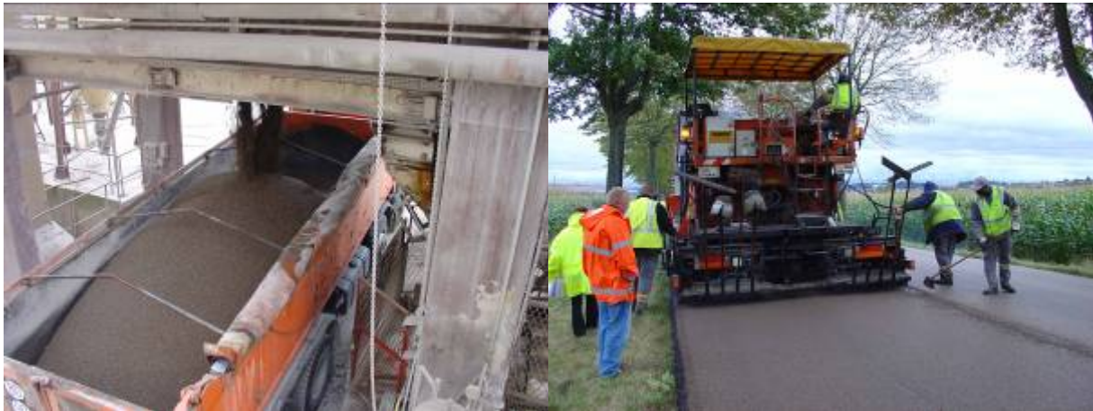
Photo 8 and 9 – loading a truck at a plant and application of the same mix on a heavily-trafficked country road.
