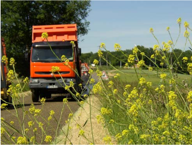
Photo 4: surface dressing in the Indre region of central France in June 2006.
