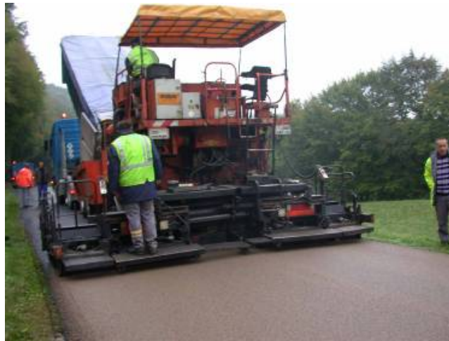
Photo 11 - October 2003, application of 0/6 asphalt mix in Ligsdorf.
