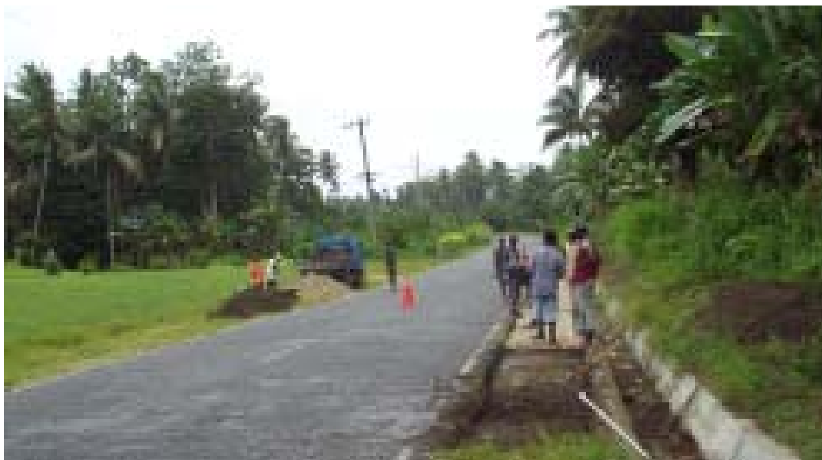
Figure 2 - Road Construction Works in Progress in Papua New Guinea.
